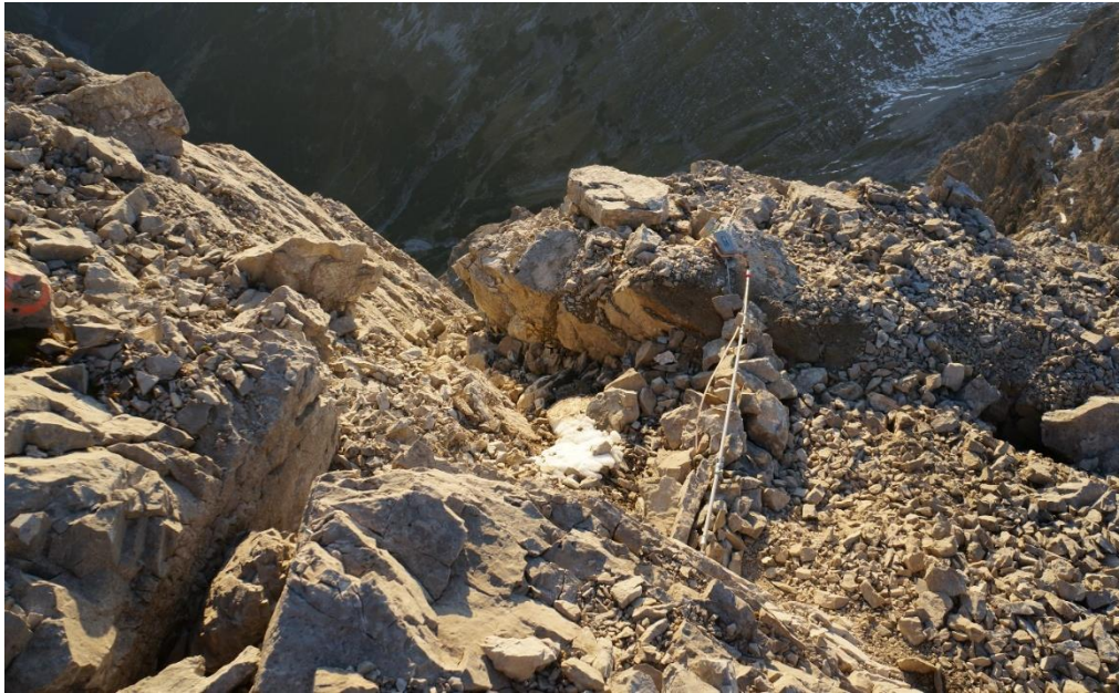
Fig. S 1: Photo of vibrating wire crackmeter "Crack06" without its protective wood roof.
