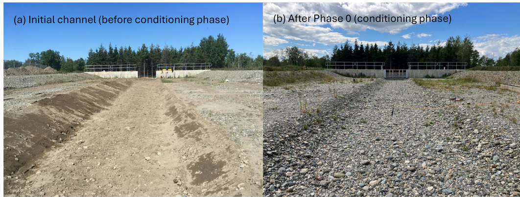
Figure 6. Oblique photographs of the straight channel showing channel adjustment under the conditioning run (phase 0). (a) Initial condition after construction, prior to water-working. (b) After the Phase 0 conditioning run (90 h), showing rapid bed-surface coarsening and development of the armour layer.
