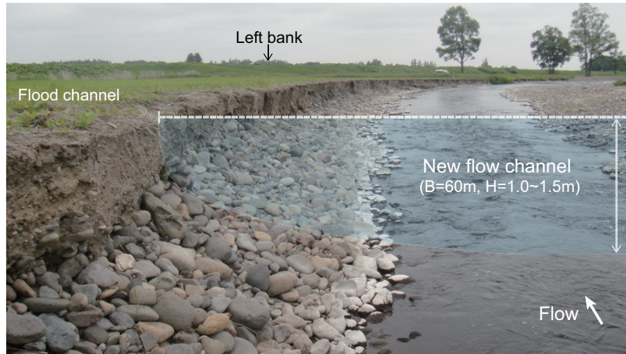
Fig. 20. New flow channel caused by the chute cutoffs in M-2.
