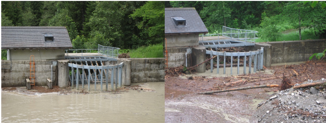
Fig. 1: Pictures of the retention basin after the flood event from the 4 th July 2009 (on the left, picture taken on the 4 th July 2009) with a peak discharge of 4990 l/s (upper gauge, 1-min. data), and after the flood event from the 20 th June 2007 (on the right, picture taken on the 21 st June 2007) with a peak discharge of 14560 l/s (lower gauge – the upper gauge malfunctioned in this event, 1-min. data).
