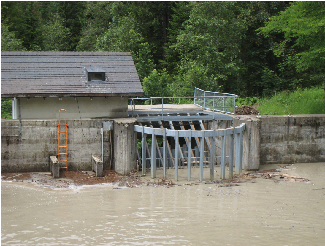
Fig. 1. Pictures of the retention basin after the flood event from the 4th July 2009 (on the left, picture taken on the 4th July 2009) with a peak discharge of 4990 l/s (upper gauge, 1-min. data).
