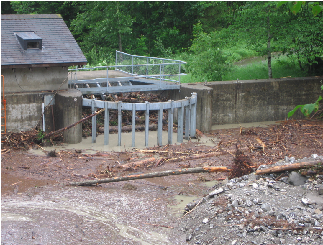
Fig. 2. Picture of the retention basin after the flood event from the 20th June 2007 (on the right, picture taken on the 21st June 2007) with a peak discharge of 14560 l/s (lower gauge).
