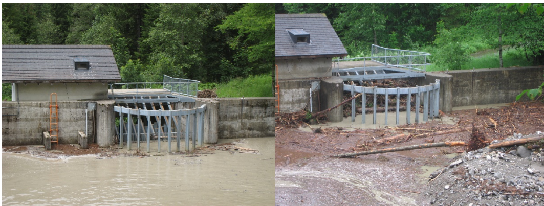
Fig. 2: Pictures of the retention basin after the flood event from the 4 th July 2009 (on the left, picture taken on the 4 th July 2009) with a peak discharge of 4990 \text{ l/s} (upper gauge, 1-min. data), and after the flood event from the 20 th June 2007 (on the right, picture taken on the 21 st June 2007) with a peak discharge of 14560 \text{ l/s} (lower gauge – the upper gauge malfunctioned in this event, 1-min. data).
