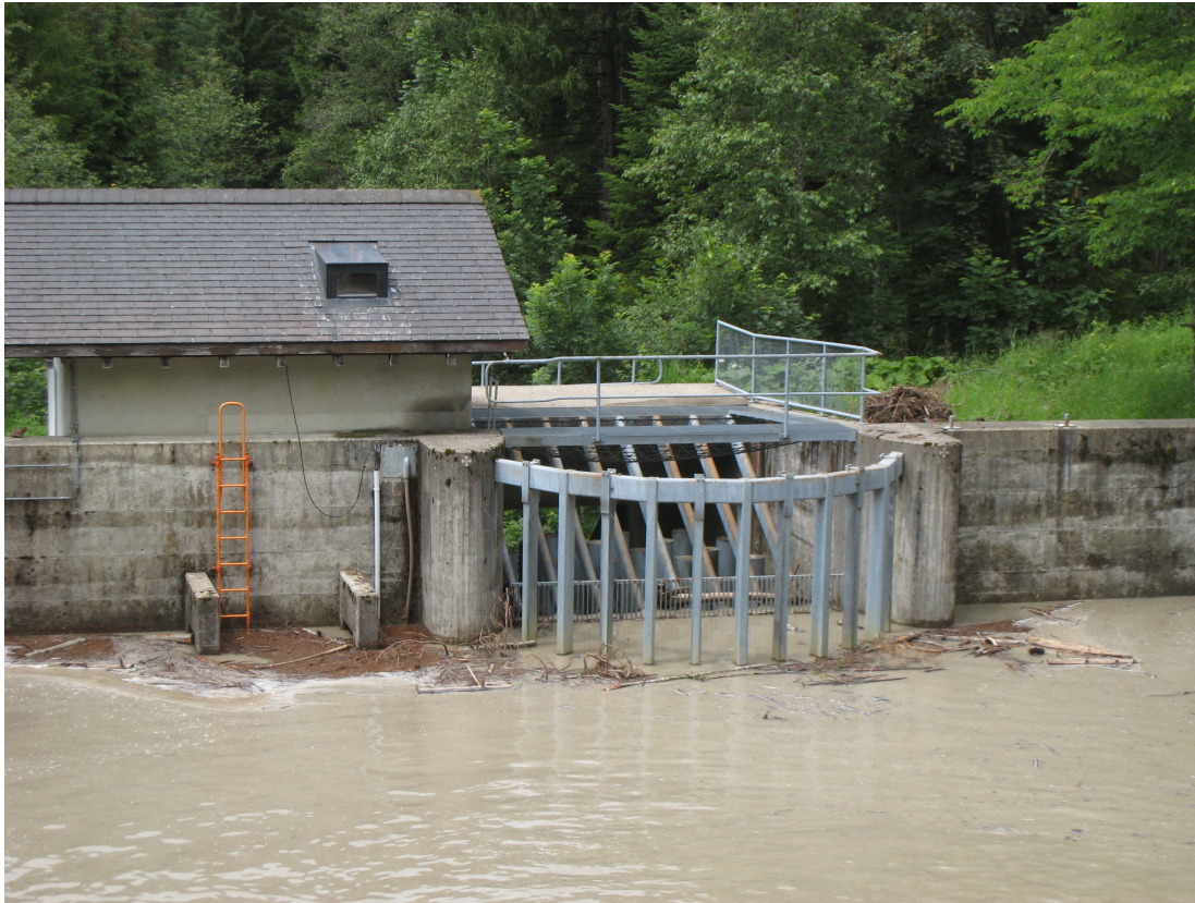
Fig. 2. Picture of the retention basin after the flood event from the 4th July 2009 (on the left, picture taken on the 4th July 2009) with a peak discharge of 4990 l/s (upper gauge, 1-min. data).
