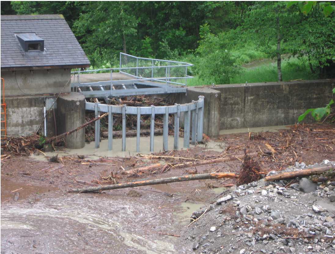
Fig. 3. Picture of the retention basin after the flood event from the 20th June 2007 (on the right, picture taken on the 21st June 2007) with a peak discharge of 14560 l/s (lower gauge).
