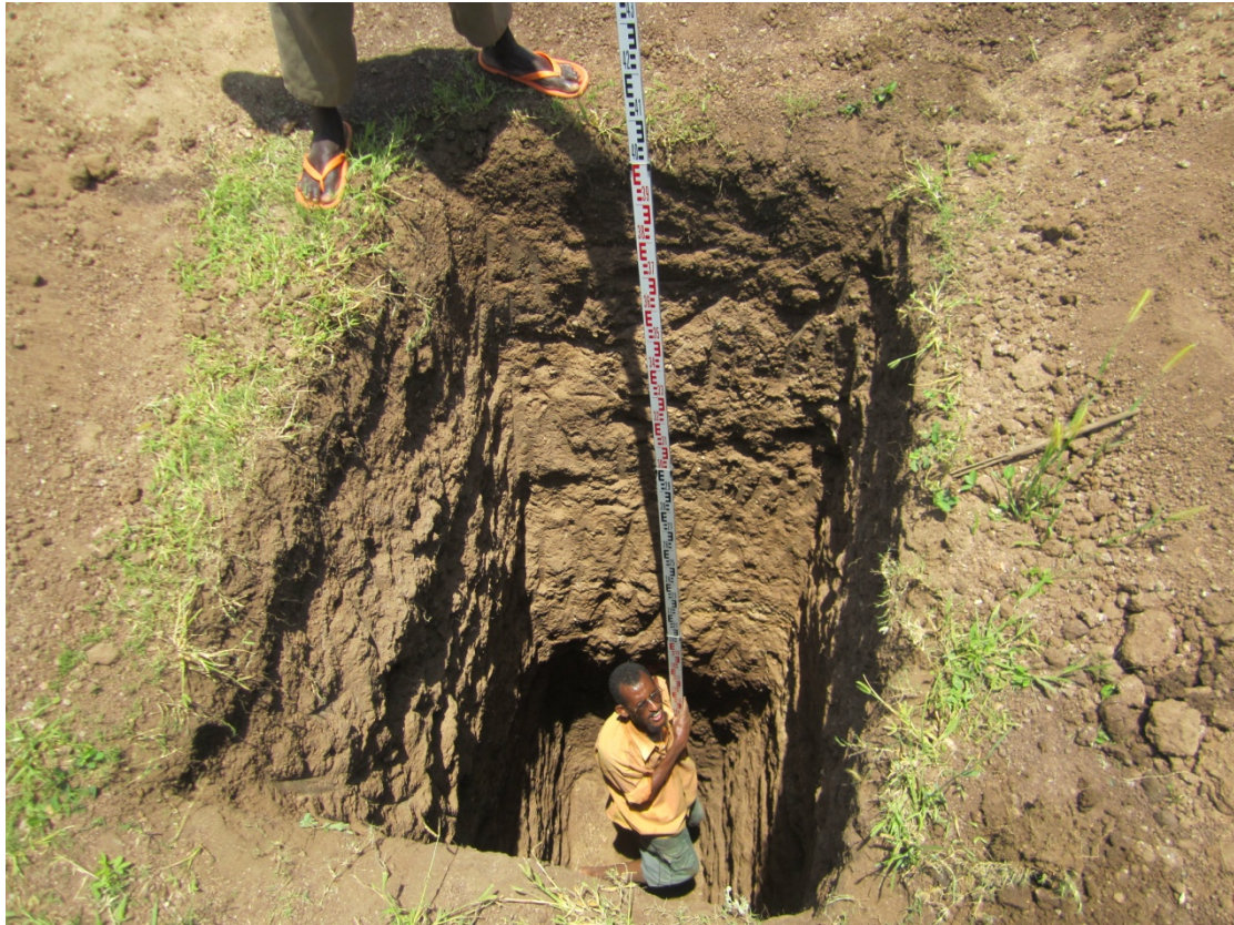
Fig. 13. Trench excavation inside Roseires Reservoir.
