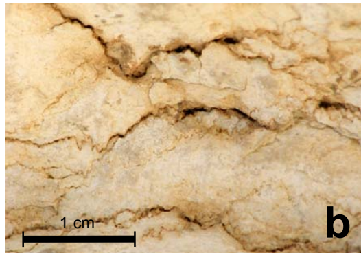
Figure 5. (a) A section of the Western Wall showing enhanced weathering in a block of micritic limestone containing stylolites. (b) Close up of a limestone block with stylolites. The millimeter-scale gaps between the seams may be indicative of mechanical particle detachment.
