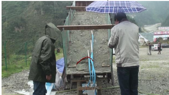
(a) Shearing opening appears in slope foot
