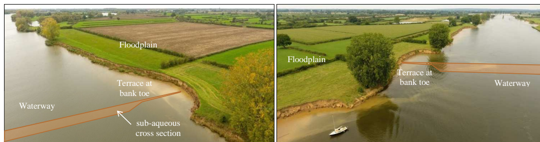
Figure 2: Restored bank in the Meuse River, upstream view of first 300 m (left) and downstream view of middle 500 m (right). Bank erosion has caused a series of bays in the 1,200 meter restored reach. Note eroded bank sediment in suspension.
