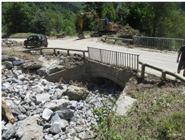
Figure 2: Effect of a sediment pulse at a bridge section of the Ruisseau de la Gorge (France), a stream that was known by local engineers for having been inactive for decades. The transported material was much finer ( D_{50} = 96 \text{ mm} , D_{84} = 169 \text{ mm} ) than the bed in place ( D_{50} = 250 \text{ mm} , D_{84} = 413 \text{ mm} ).
