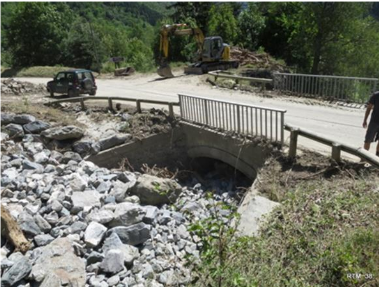
Figure 2: Effect of a sediment pulse at a bridge section of the Ruisseau de la Gorge (France), a stream that was known by local engineers for having been inactive for decades. The transported material was much finer ( D_{50} = 96 \text{ mm} , D_{84} = 169 \text{ mm} ) than the bed in place ( D_{50} = 250 \text{ mm} , D_{84} = 413 \text{ mm} ).
