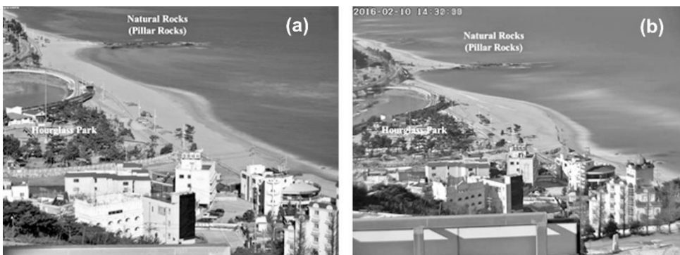
Figure 2: Beach erosion at Jeongdongjin Beach, South Korea caused by (a) low waves on 04 December 2015 and (b) high waves on 10 February 2016.
