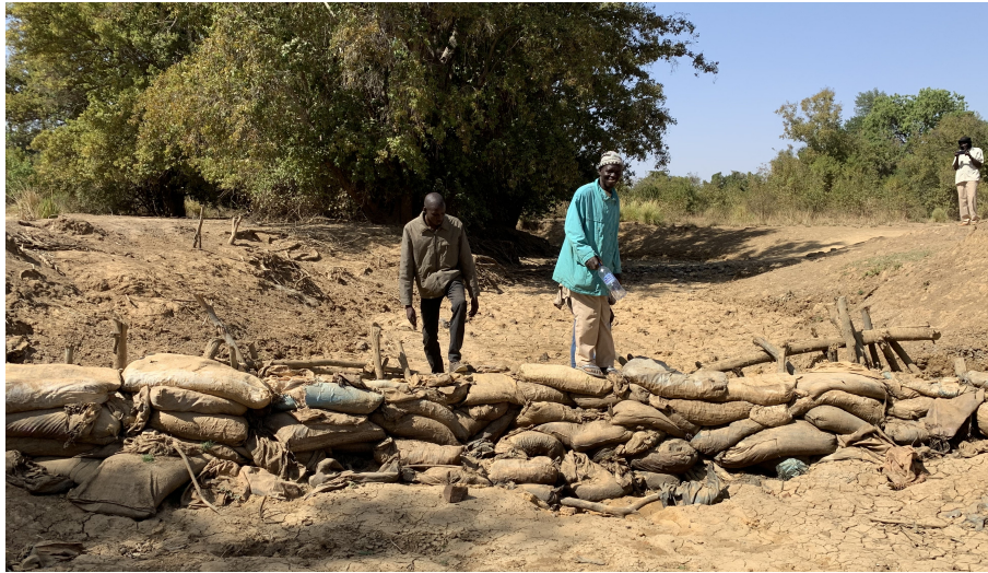
Figure 13. Photo of the hand-made dam at the outlet of Lac Wégnia (9 February 2020, Source: Tobias Siegfried).
