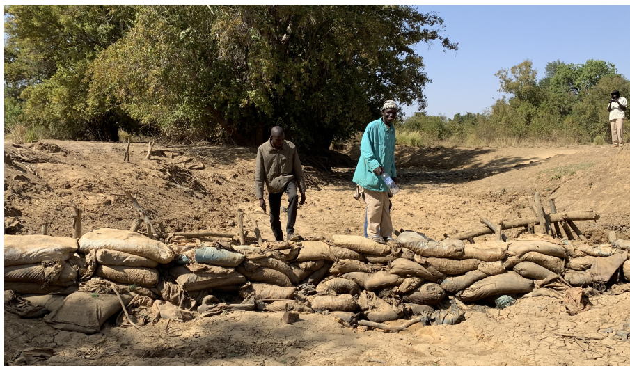
Figure 13. Photo of the hand-made dam at the outlet of Lac Wégna (9 February 2020, Source: Tobias Siegfried).
