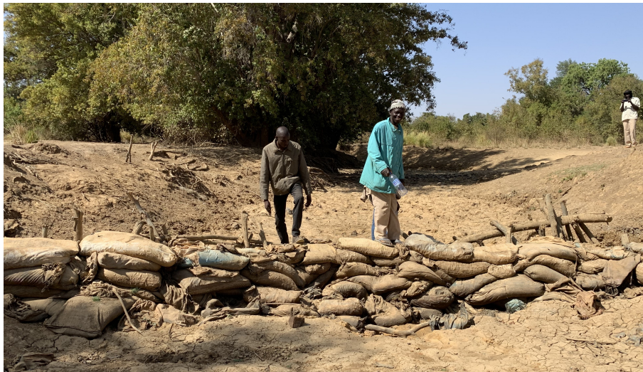
Figure 13. Photo of the hand-made dam at the outlet of Lac Wégניה (9 February 2020, Source: Tobias Siegfried).
