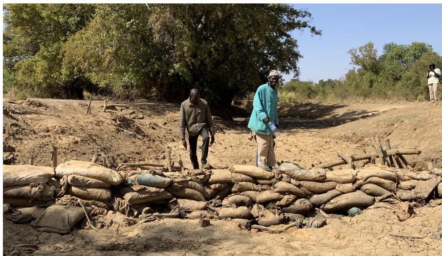
Figure 13. Photo of the hand-made dam at the outlet of Lac Wégניה (9 February 2020, Source: Tobias Siegfried).
