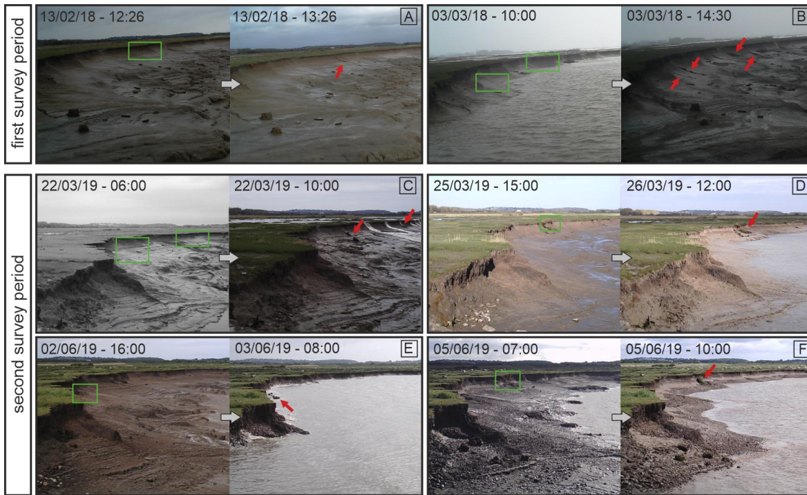
200 Figure 4. Time sequences of notable mass failure events identified at the study site during the two periods of deployment of the fixed camera. Red arrows in the photographs indicate the collapse events; green boxes highlight the site of the bank where successive collapses occur. Photographs connected by white arrows are successive (very close) in time. The failure events are also highlighted in the tidal range charts in Figure 3.
