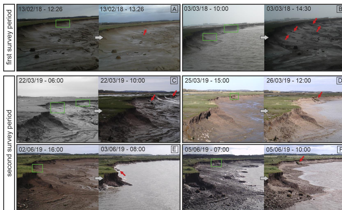
175 Figure 4. Time sequences of notable mass failure events identified at the study site during the two periods of deployment of the fixed camera. Red arrows in the photographs indicate the collapse events; green boxes highlight the site of the bank where successive collapses occur. Photographs connected by white arrows are successive (very close) in time. The failure events are also highlighted in the tidal range charts in Figure 3.
