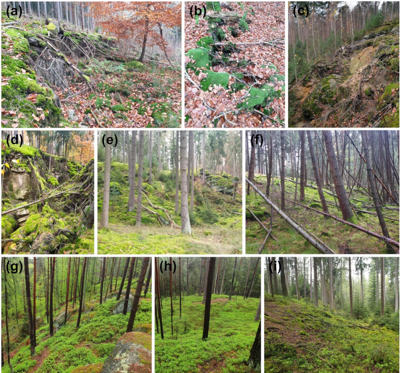
Figure 34: Photos of (a-b) lateral roots under tension located at the headscarp and (c) at a secondary scarp of the Putzenstein landslide. (d) Rhätolias boulders at the headscarp, (e) overview of the headscarp and (f) tilted trees at the toe of the Weinreichsgrab landslide. (g-h) Overview about the headscarp and (i) the toe of the Fürstenanger landslide.
