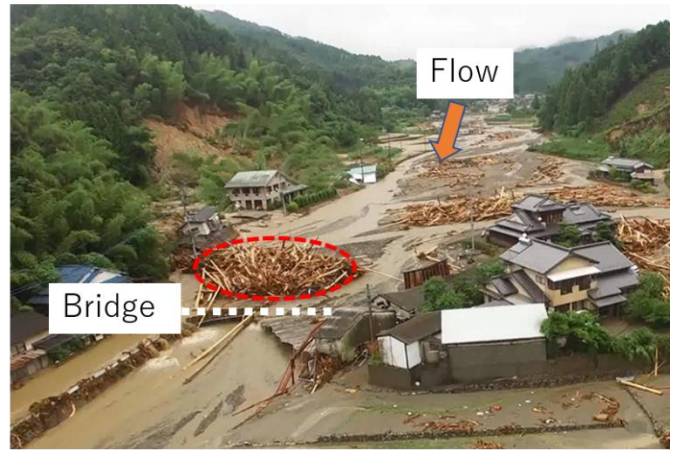
Figure 1: Large wood deposition at the outlet of a valley bottom (left) and large wood depositions at around the bridges (right) in the Akatani river flood disaster, 2017.
