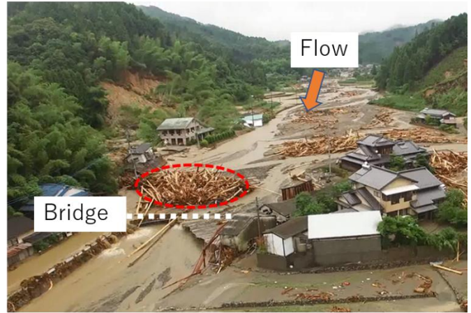
385 Figure 1: Large wood deposition at the outlet of a valley bottom (left) and large wood depositions at around the bridges (right) in the Akatani river flood disaster, 2017.
